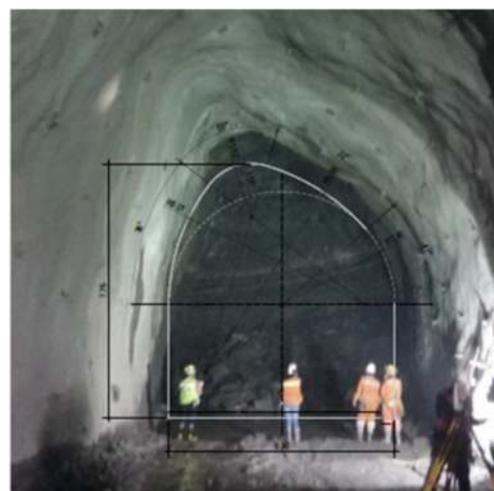
Figure 2: Initial modification of the excavation shape by Contractor to follow the failure mode (7.35 m of vertical dimension)
