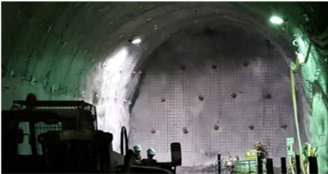
Figure 11: Examples of application of the Double-layer solution and tunnel face control
