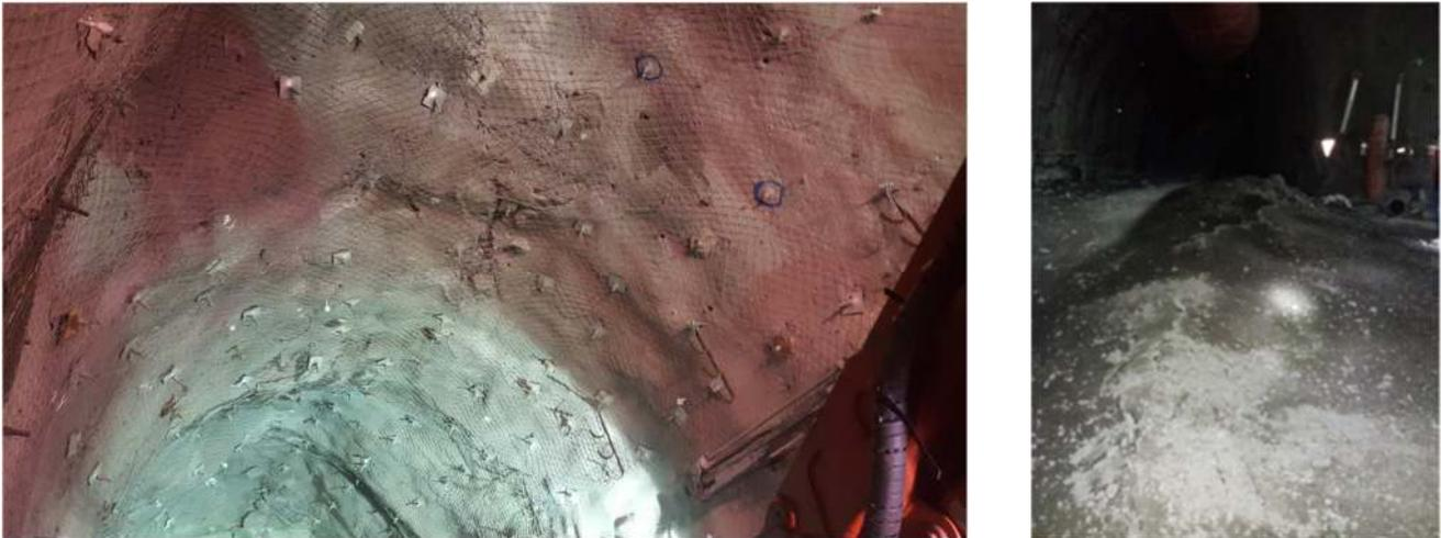
Figure 15. Examples of damage of the support systems in crown and invert for severe rockburst events
