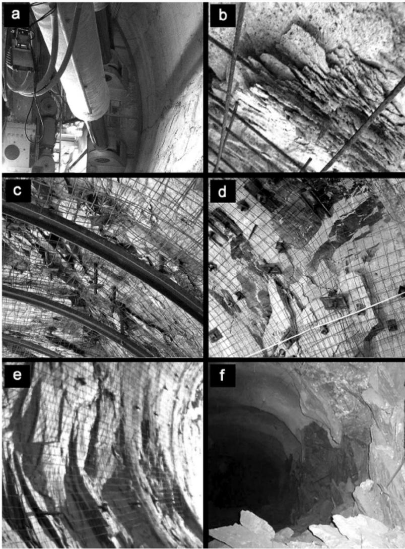
a→f=increasing levels of spall damage
