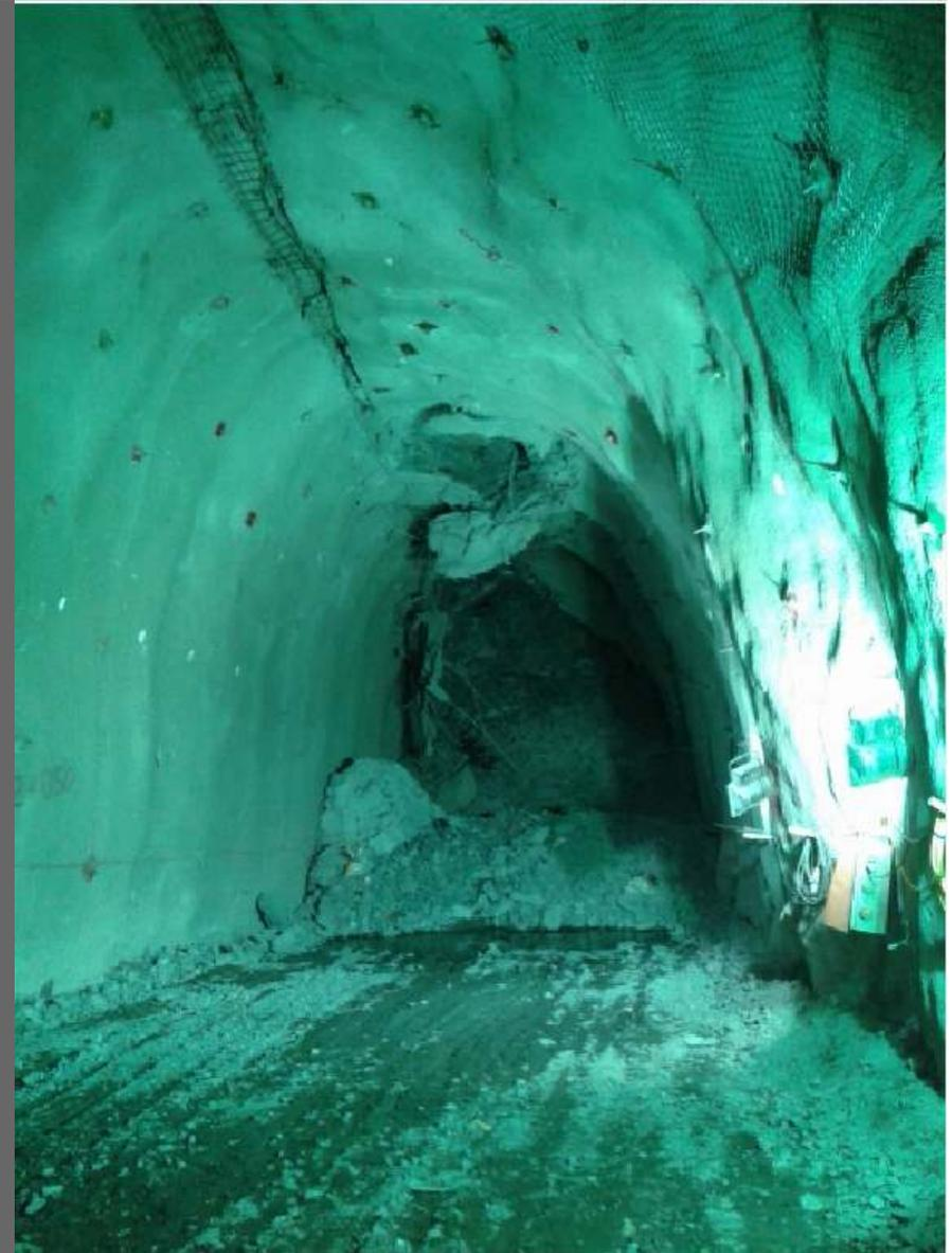
**Example of DISL application in severe rockburst environment**
