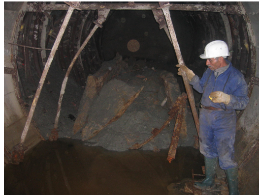
Fig.5: Failure of the invert for swelling behaviour of clayey flysch in the experimental Malabata well on Moroccan coast of the Gibraltar strait
