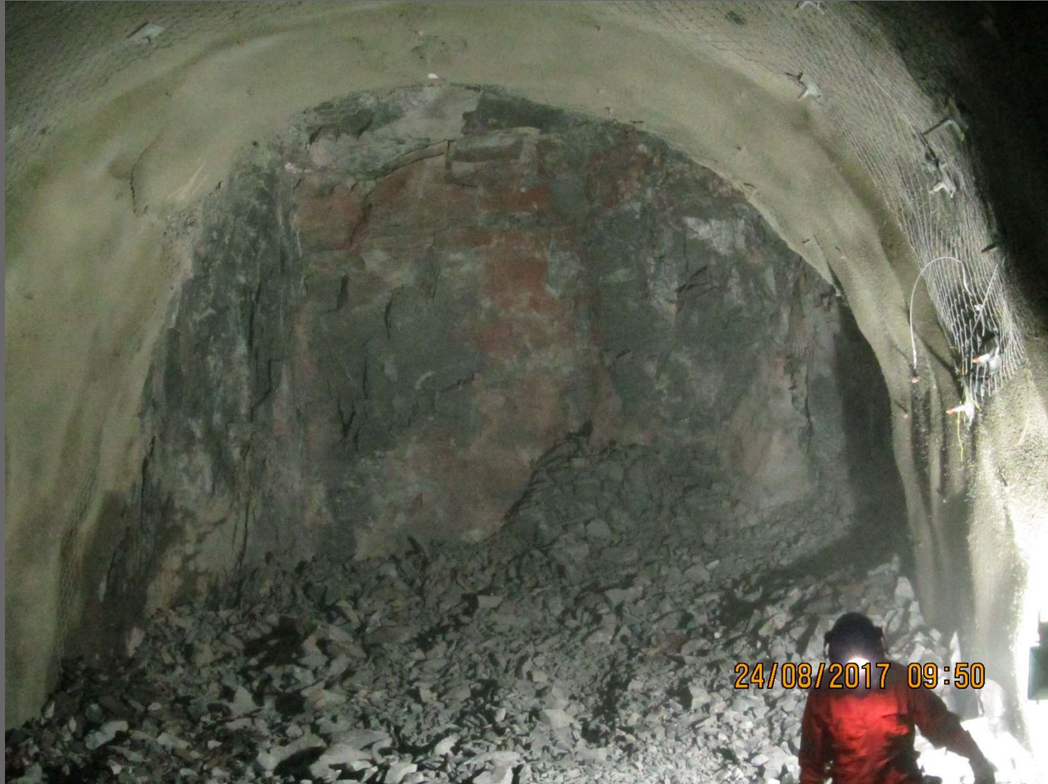
Some laminated shear bands in the adit face
