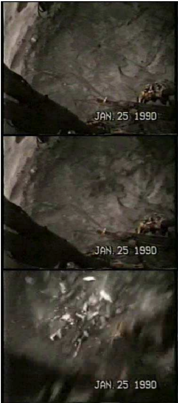
Fig. 3.3: The dramatic sequence of heavy rock-burst occurred in the Maule Tunnel (Chile) during drilling. The tunnel was crossing hard grain-diorites with overburden of about 1000m (→case-history ch5). Note in the central photogram, the development of fracturing in the upper right part of the tunnel face. The elapsed time between the first and third photogram is less than 1sec (Video: courtesy of F.A. Anadon (Dragados))
