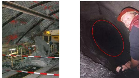
Fig.2.1: Example of rockburst (left: Loetschberg Tunnel, Diederichs, 2005) and squeezing behaviour (right: deformation in the pilot tunnel of the Fleres railway tunnel excavated by TBM)
