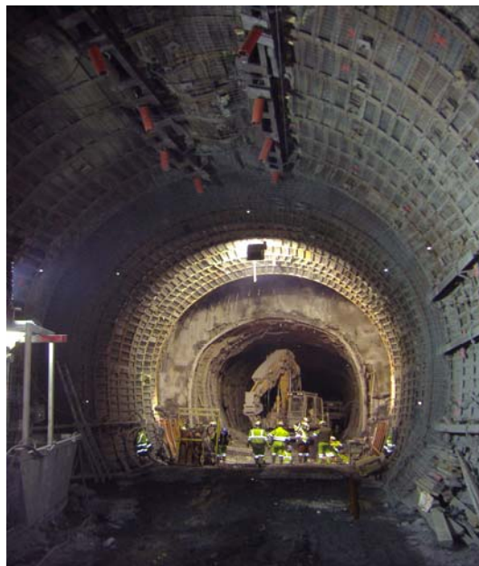
Figure 4. Image of the deformed excavation section and of the enlarged one after re-shaping.
